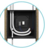
Install drainpipe, linesets, high/low voltage wiring.
